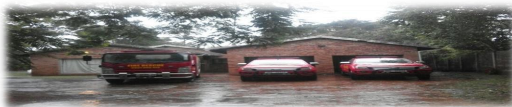
Figure 3. uMfolozi Disaster Management Fire and Rescue base in Kwa-Mbonambi
