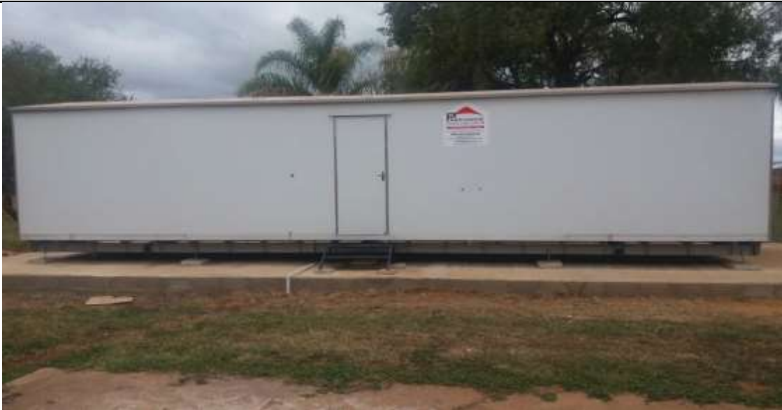
Figure 63: Disaster Management Building
