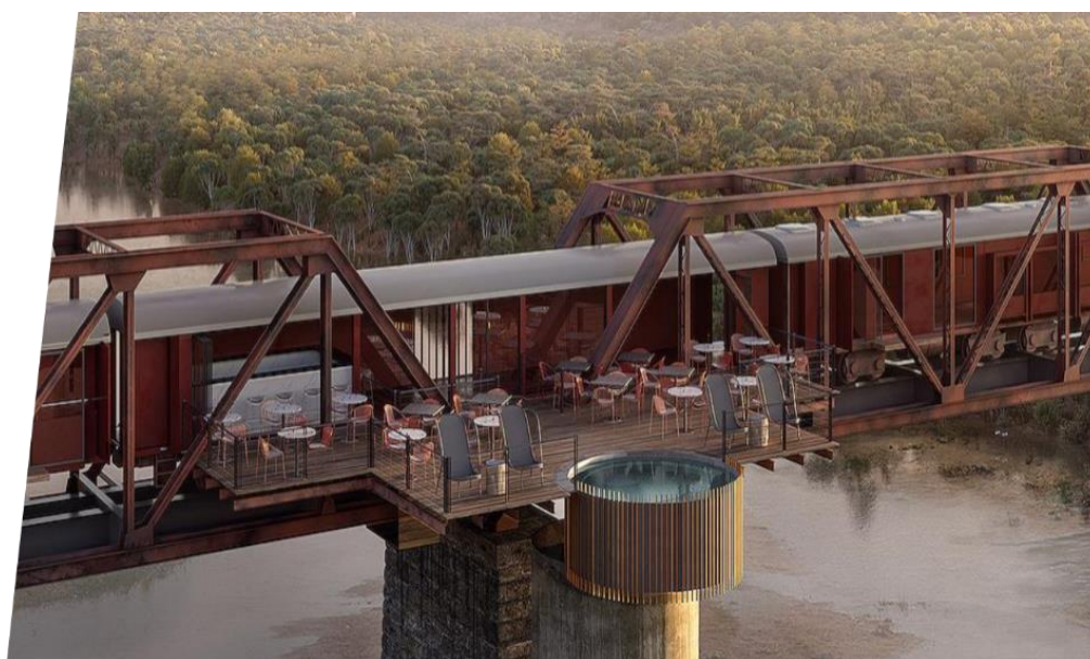
Figure 50: Kruger Shalati (The Train On The Bridge)
