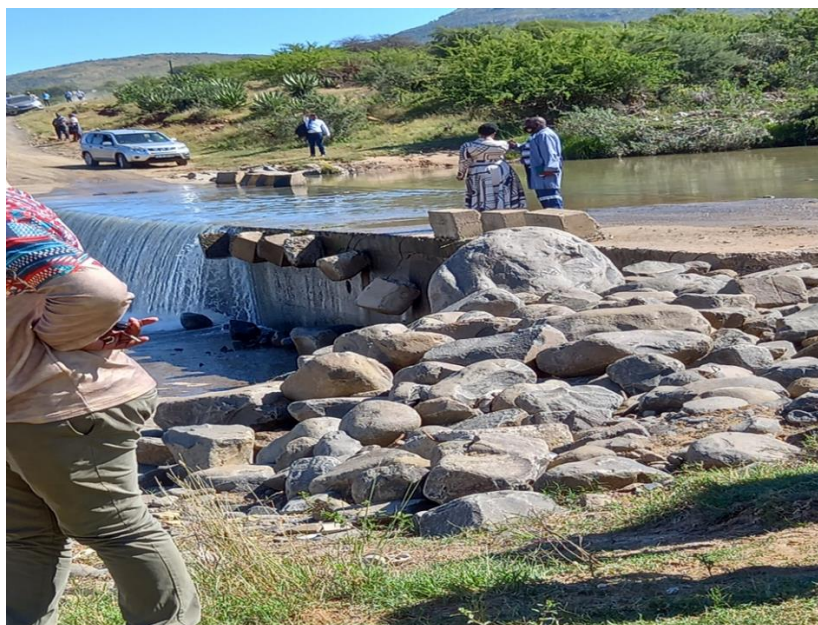
FIGURE 31: LOW-LYING BRIDGE AT SAMPOFU AREA, WARD 17
