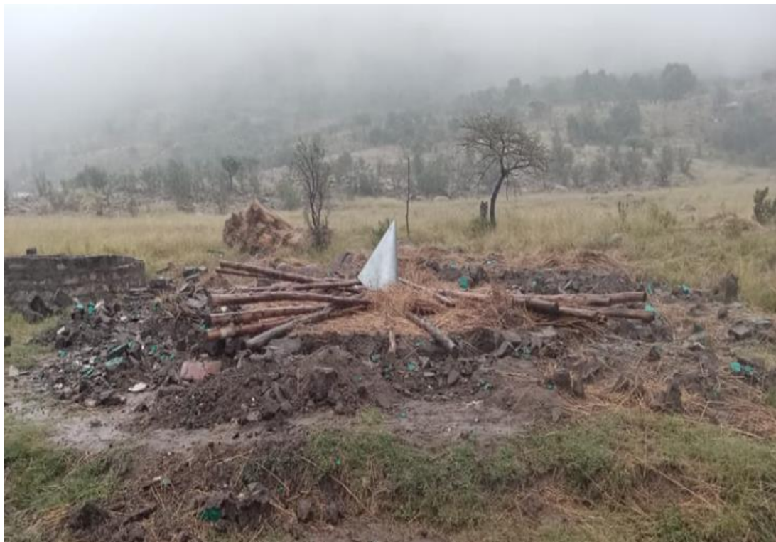
FIGURE 29: HOUSES DAMAGED AT WARD 4 AT ESIDAKENI
