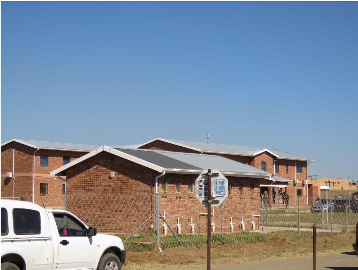
Visual 13: New Nquthu Traffic Offices and Testing Grounds was officially opened on 22 May 2024.
