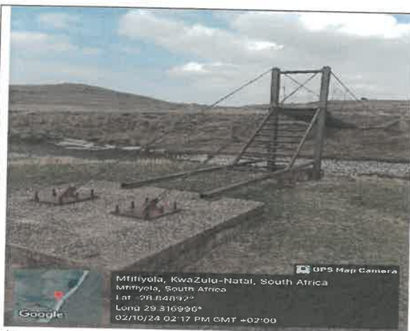
Figure 3 Ngoba steel pedestrian bridge.
