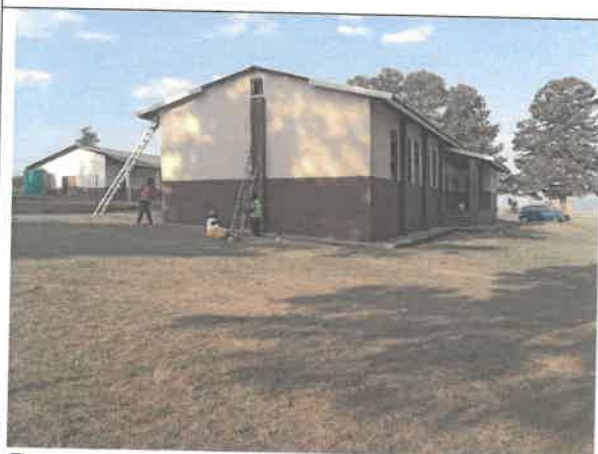
Figure 4; Renovations at Zwelisha community hall.
