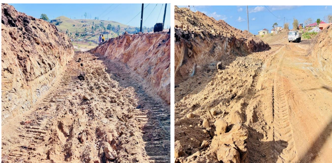
Photos: LIC Road Construction (Mgorha road, ward 09)
