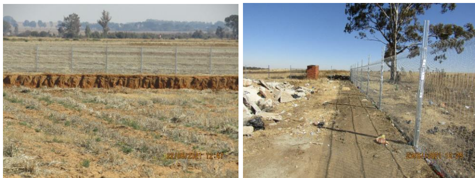
Figure 2: Excavation of the pollution dam at Viljoenskroon Landfill Site and the fencing of the Steynsrus Landfill Site.
