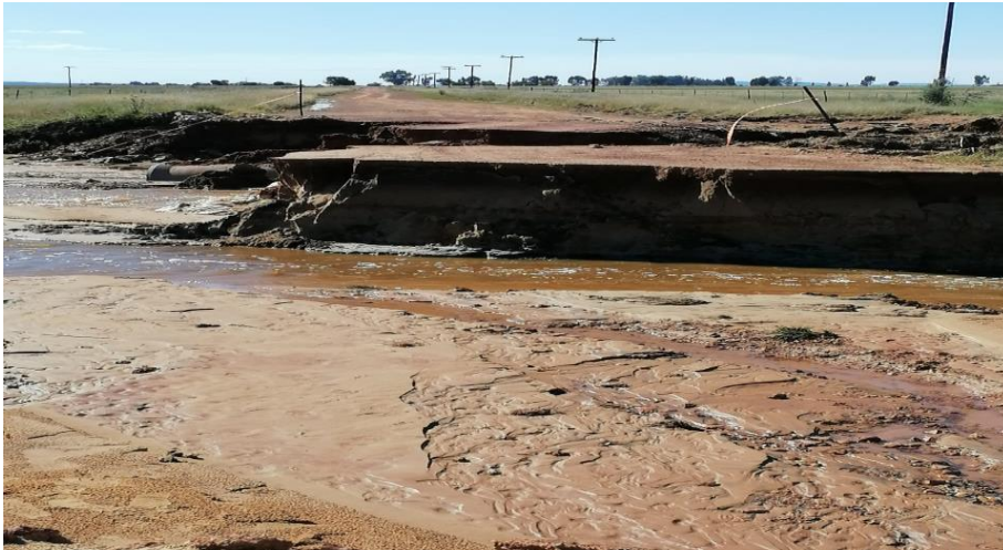
Figure 7 Eroded Road
