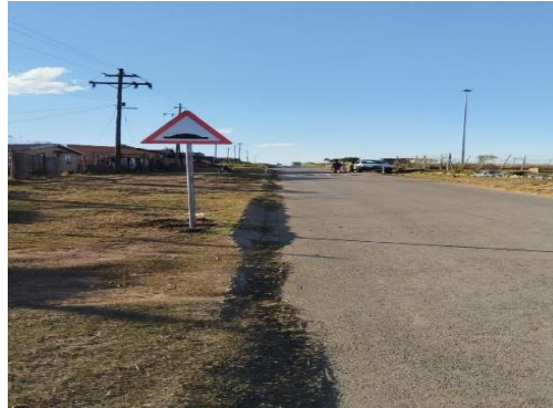
Picture 22: Installation of road sign
