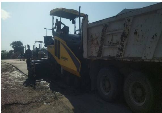
Picture 19: Resurfacing of roads in progress
