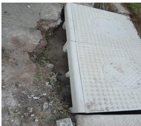
Picture 26: Installation of Stormwater Manhole cover
