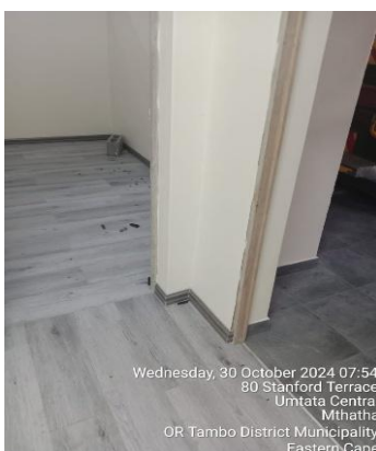
New floor covering
