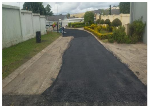
Picture 18: Pothole Patching Completion
