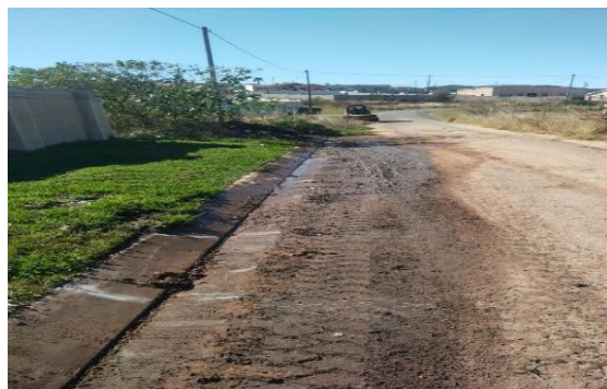
Picture 24: Unblocking Stormwater Drainage Picture 25: Cleaning Stormwater Channel
