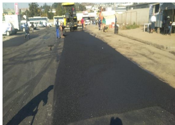
Picture 20: Resurfacing of roads completed
