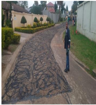
Picture 17: Pothole Patching Preparation
