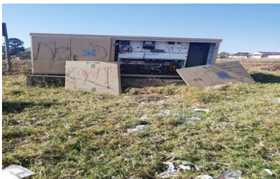
Picture 4: Vandalized Mini Substation
