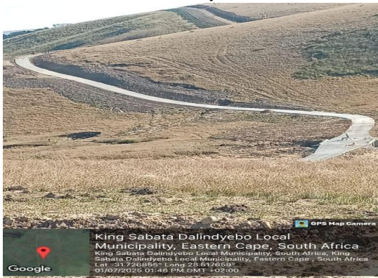
Picture 5: Mkwezo to Mpandela Concrete Road
