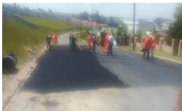
Picture 11: Resurfacing of roads in progress
