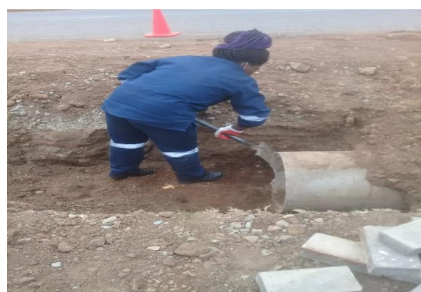
Picture 10: Unblocking Stormwater Drainage
