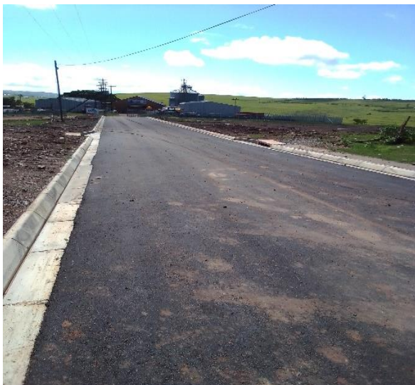
Picture 3: Viggies to Sawmill Road Surfacing
