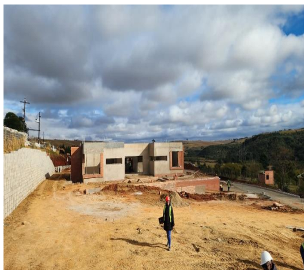
Picture 4: Mqanduli DLTC under Construction
