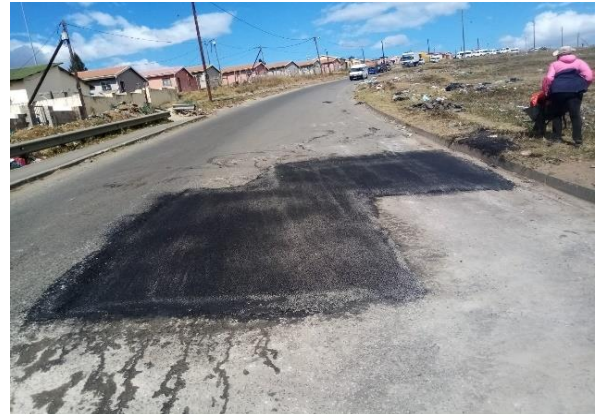
Picture 8: Pothole Patching Completion
