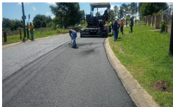
Picture 12: Resurfacing of roads completed
