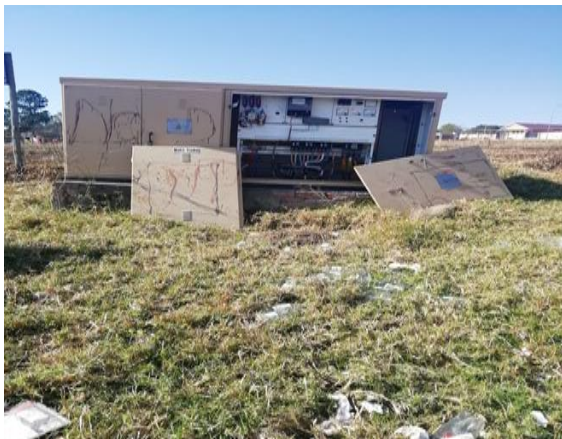
Picture 16: Vandalized Mini Substation
