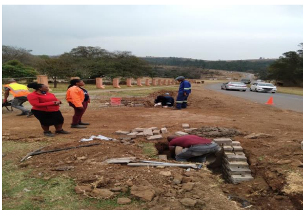
Picture 9: Manhole repairs
