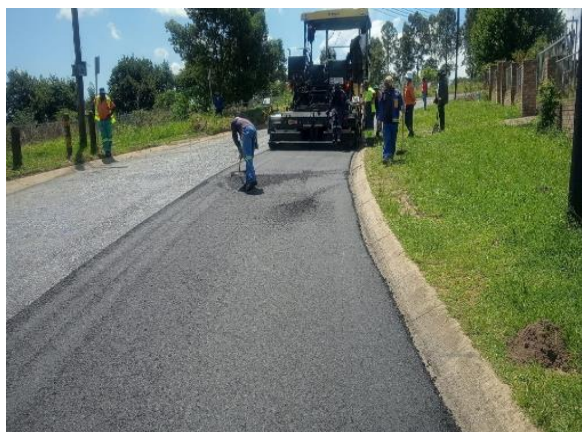
Picture 12: Resurfacing of roads completed
