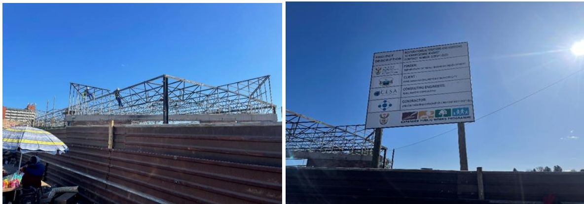
Picture 23: Roof works Construction of KwaNtozonke Market
