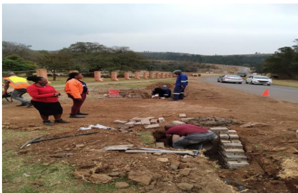
Picture 9: Manhole repairs
