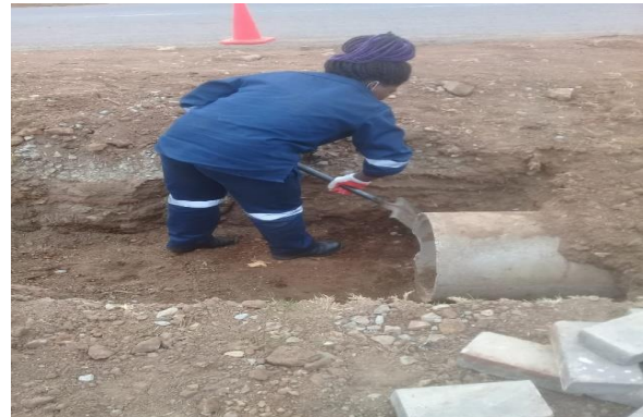
Picture 10: Unblocking Stormwater Drainage
