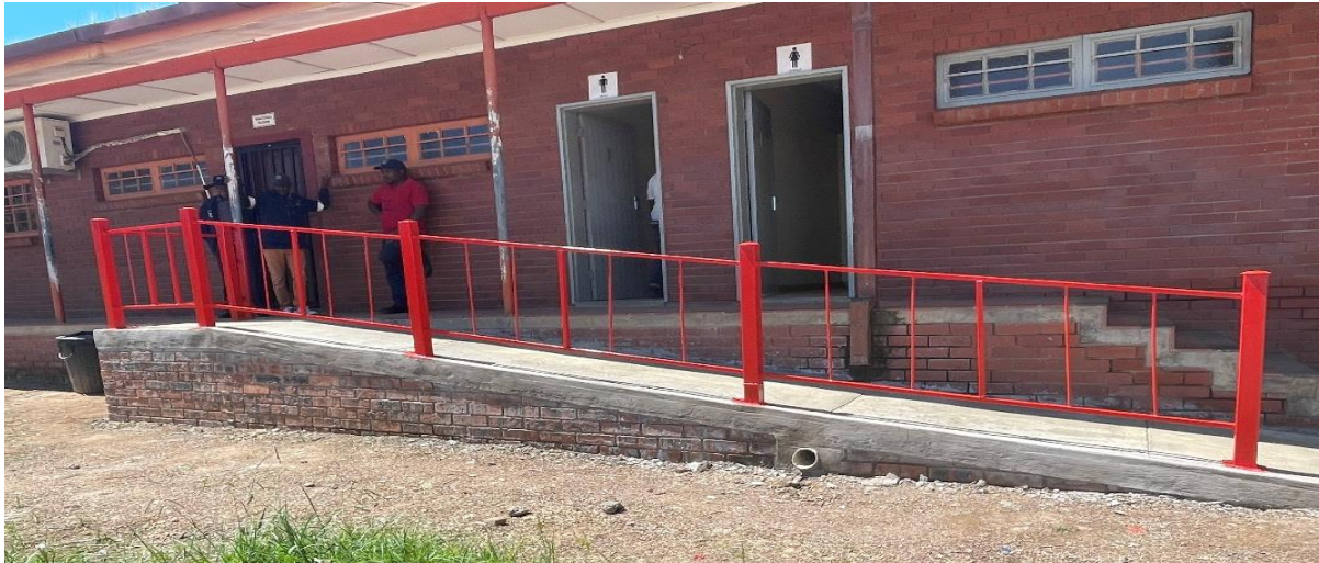
Picture 19: New constructed Ramp at DLTC
