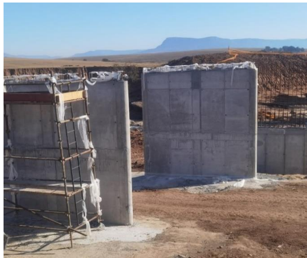
Picture 2: Baziya Bridge under Construction
