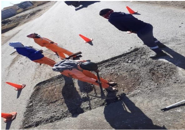
Picture 7: Pothole Patching Preparation
