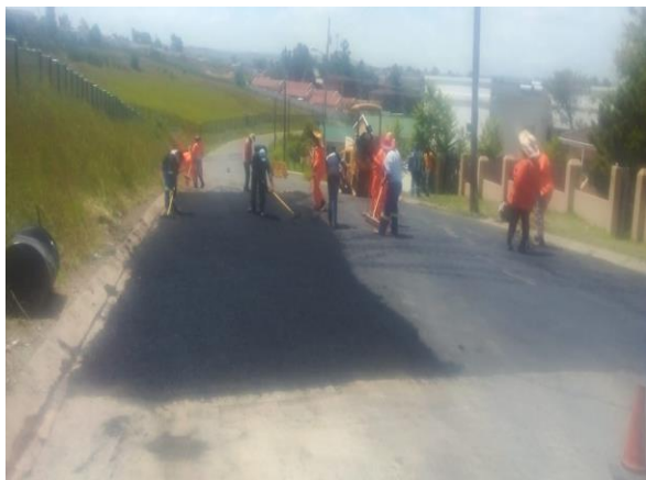
Picture 11: Resurfacing of roads in progress
