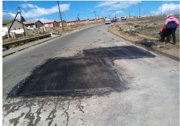
Picture 8: Pothole Patching Completion
