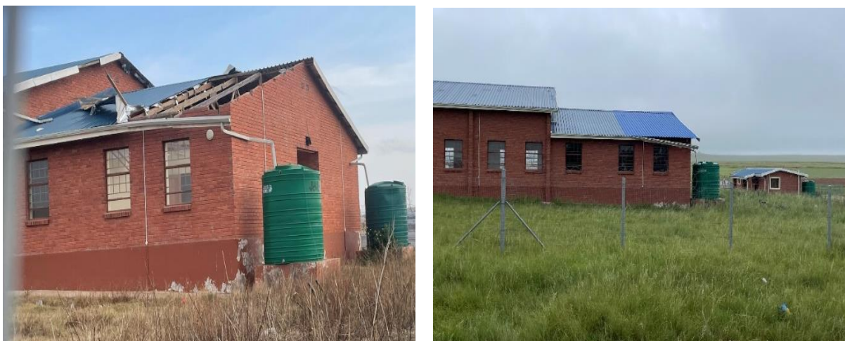
Picture 18: Maintenance of Mdeni Community Hall in Ward 34
