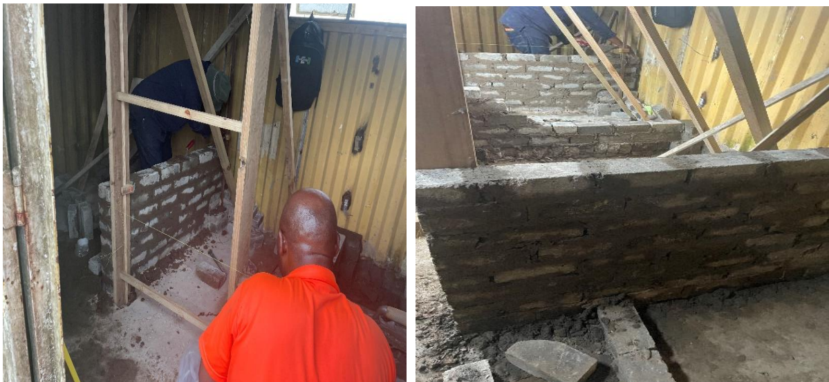
Picture 22: Construction/Partitioning of toilets for Employees at Khwezi Landfill Site
