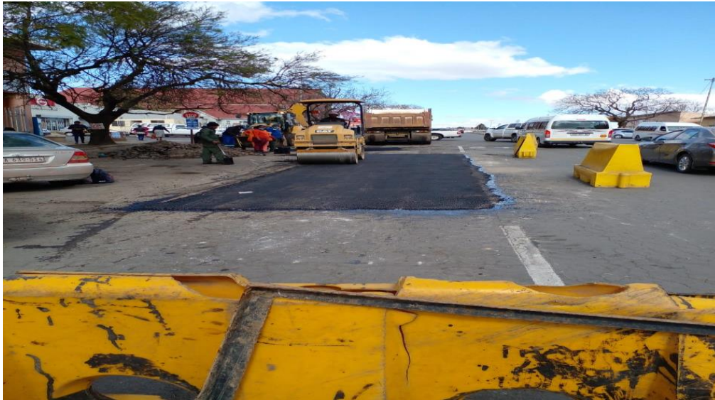
Surface street (Pothole Patching in ward 13, North crest, Jizana street.
