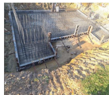
Kwanomzamo WWTW Refurbishment
