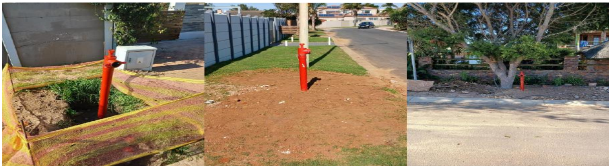
New Water Main in Mimosa Street
