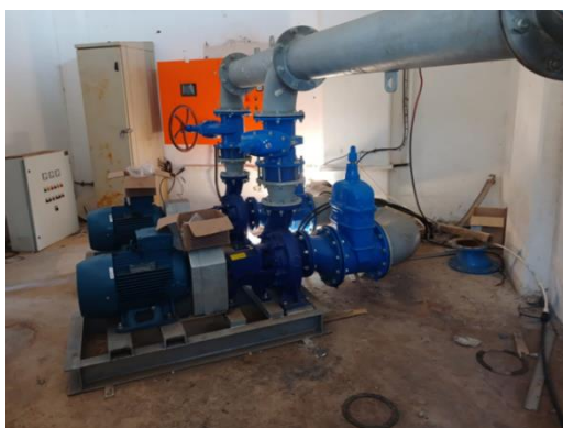
New pumps installed at the Paradise Beach Water Tower
