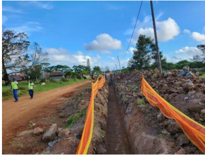
Kruisfontein Trench excavation.
