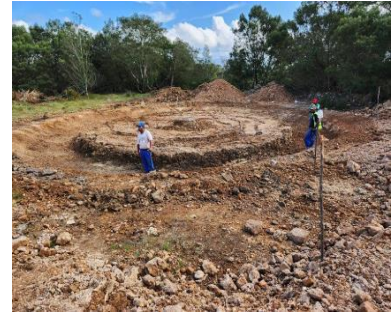
Kruisfontein: Ring beam for break pressure tank.
