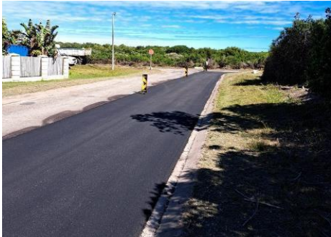
St Francis Bay: St Francis Drive reseal
