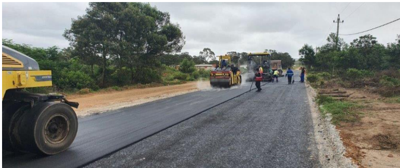
Upgrading of Gravel Roads Phase 1
