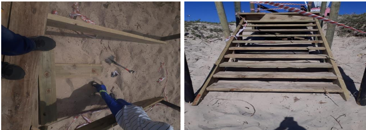
Repairing of walk way
