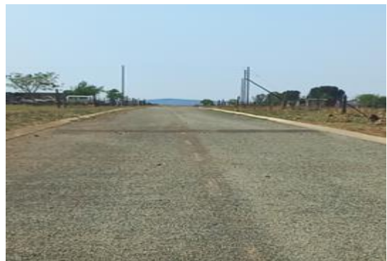
Double Sealed road
