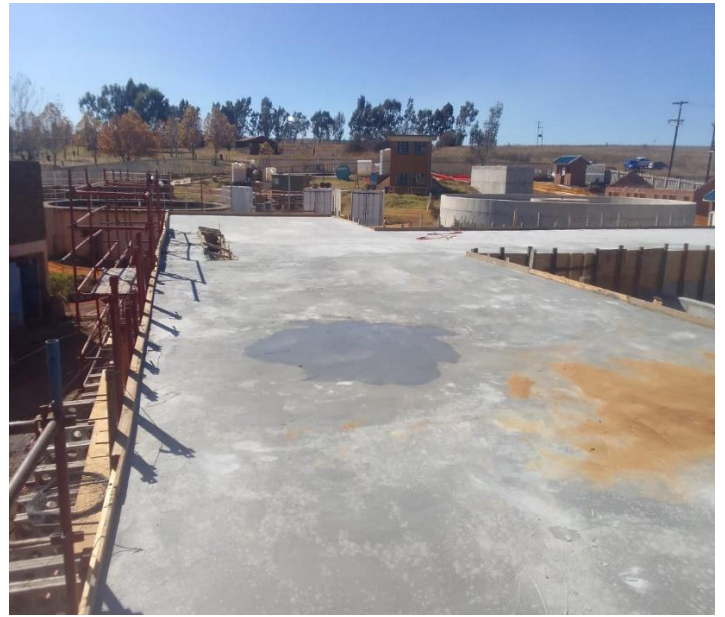
During the curing of the service building operational slab and roofing for the buildings in the Upgrading of Fortuna Water Treatment Works under Balfour/Siyathemba/ Nthorwane/Greylingstad Bulk Water Scheme
