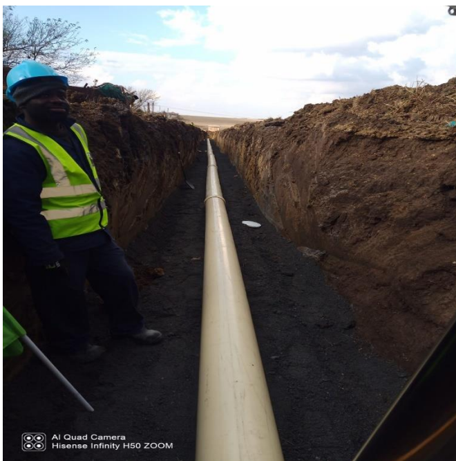
During the Construction of the gravity sewer lines 250/160 in Rooikoppen phase 1 and 4
