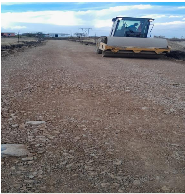
Stabilizing Layers for access road and laying of pipe in Rooikoppen in Lekwa Local Municipality
