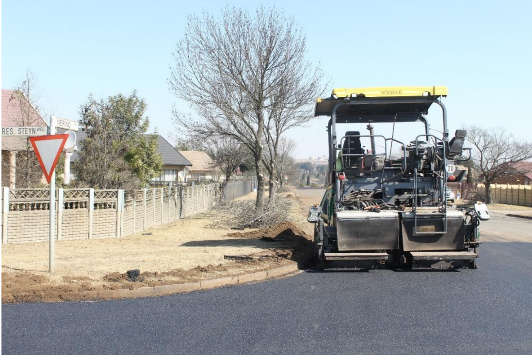
PHOTO: Road Rehabilitation Programme in Msukaligwa, 2023.
