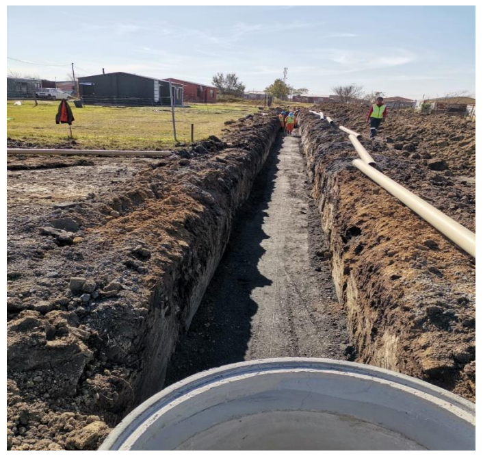
During the Construction of the gravity sewer lines 250/160 in Rooikoppen phase 1 and 4
