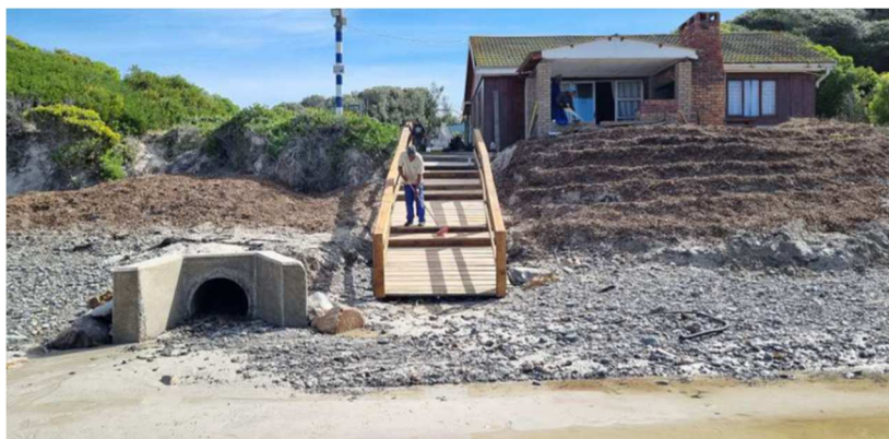
Upgrading of stormwater pipe and wooden steps at Uilenkraalsmond
