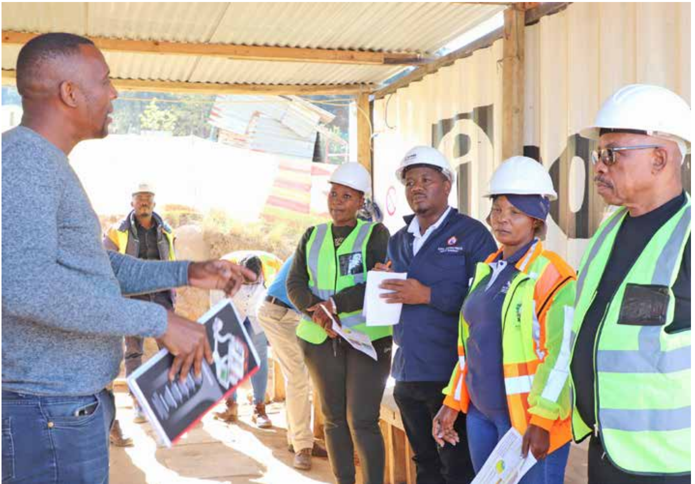
Oversight visit to monitor progress on Middledrift Water project
