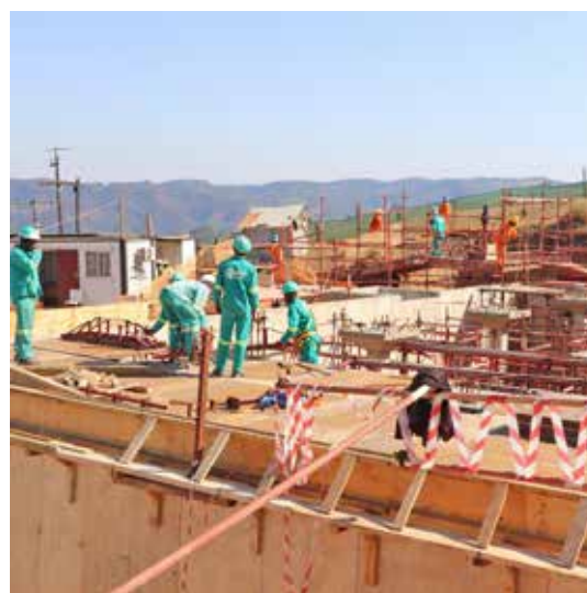
Middledrift Project under construction in August 2024
