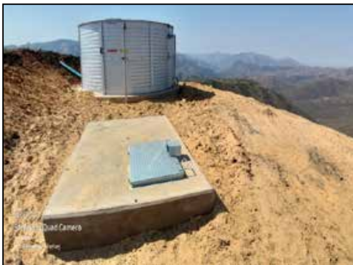
Photo 2: Air valve ring manhole
