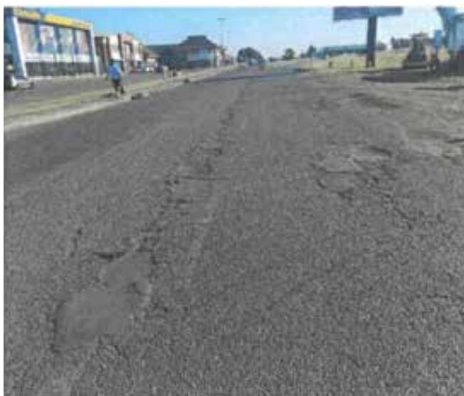
Photo 12: Road repairs before
