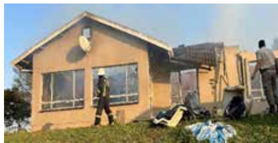
Photo 2: Totally destroyed house in Ward 11 Eshowe.
