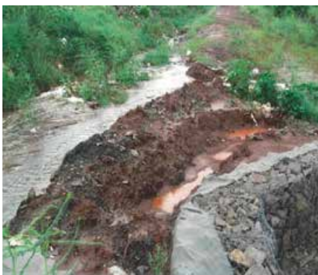
Photo 10: Road access before
