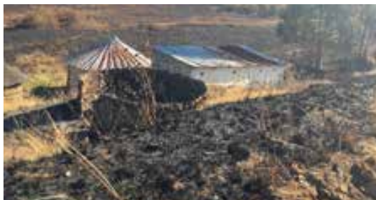
Photo 1: A house that was destroyed by Veld fire at Ward 06 Hlangana, Umlalazi.
