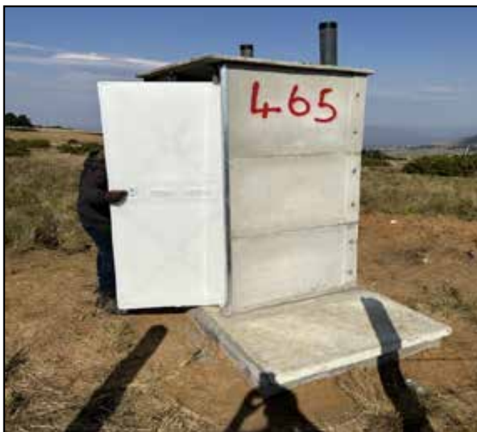
Photo 1: Completed VIP Toilet
