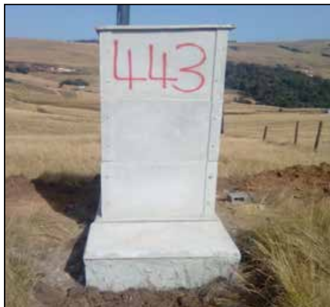
Photo 2: Completed VIP Toilet
