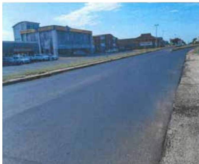
Photo 13: Road repairs after
