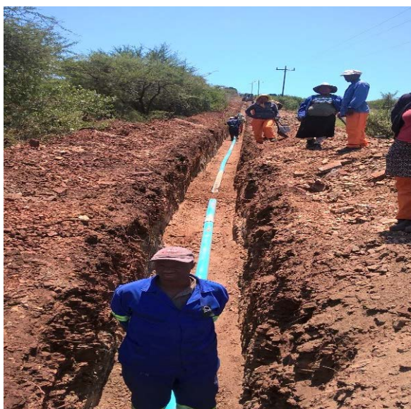
Photo 4: Laid pipe before backfilling
