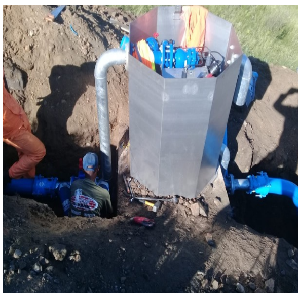
Photo 3: Installation of BPT (Break Pressure Tank)
