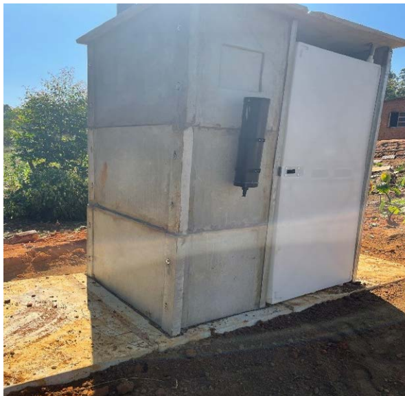
Photo 2: Completed VIP Toilet showing the complete unit with lockable door.
