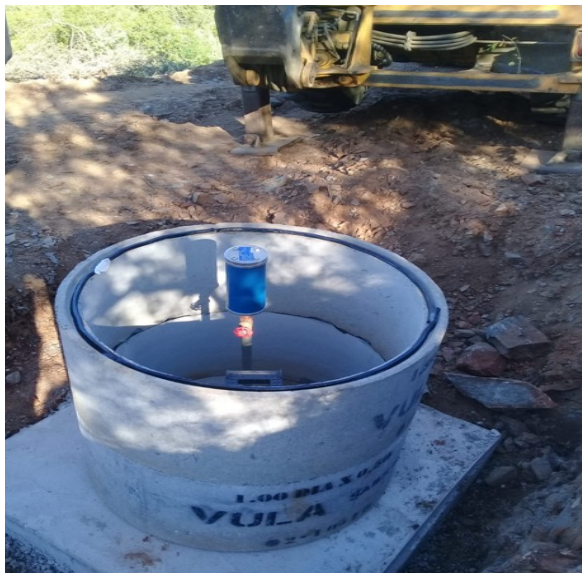
Photo 2: Construction of air valve ring manhole
