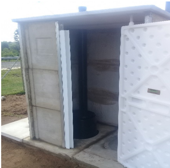
Photo 3: Completed VIP Toilet
