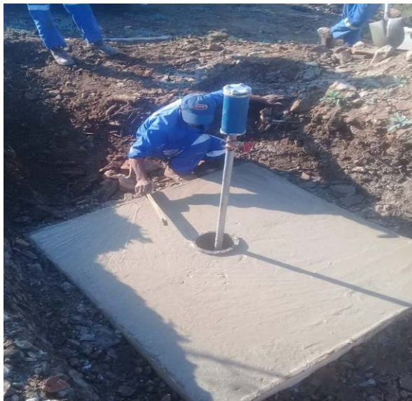
Photo 1: Casting of air valve base
