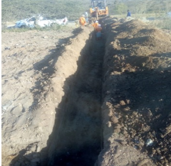
Photo 2: Excavation for Pipelaying
