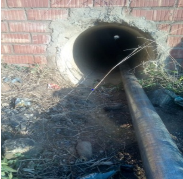
Photo 1: Main road crossing through stormwater
