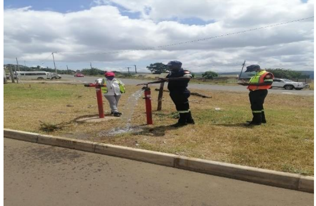
Image 2: depicting Fireman conducted water hydrant inspection at Jozini L.M
