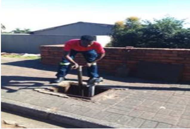
Image 1: depicting Fireman conducted water hydrant inspection at Mtubatuba L.M
