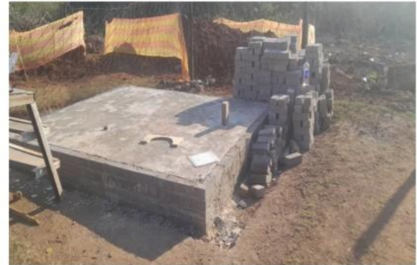
Concrete Slab- Guard Foundation
