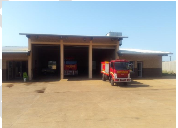
Image 2: Fire Station of UKDMC
