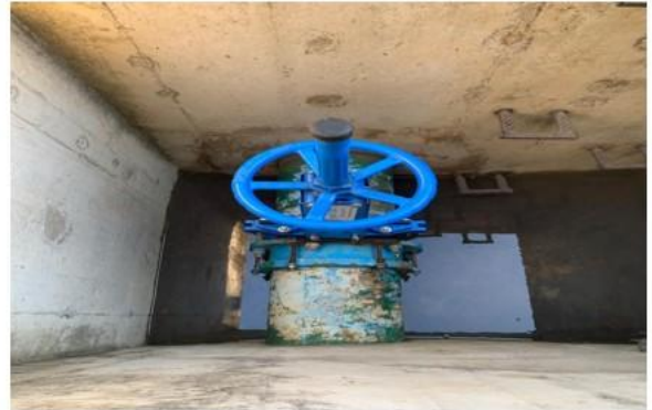
Installation of 200mm Isolation Valve
