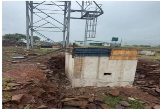
Elevated Tank Inlet Chamber
