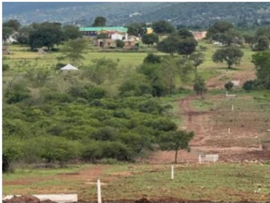
Rehabilitation along 200DN Pipeline
