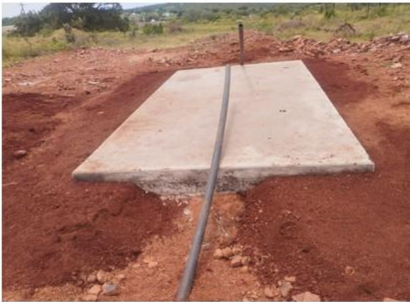
Base concrete slab
