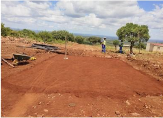
Pump base preparation
