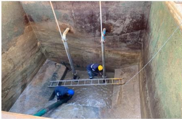
Clearing of Sludge Sump
