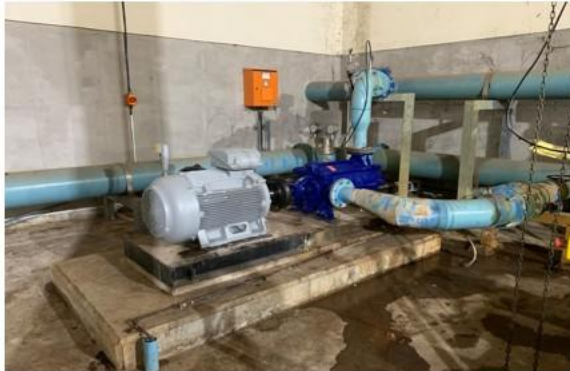
Installation High lift Pump
