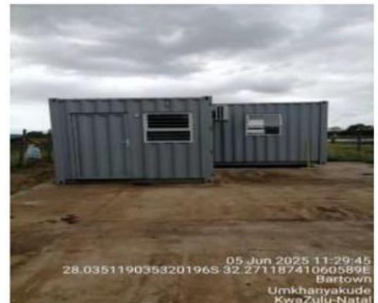
Mobile Office and Guardhouse
