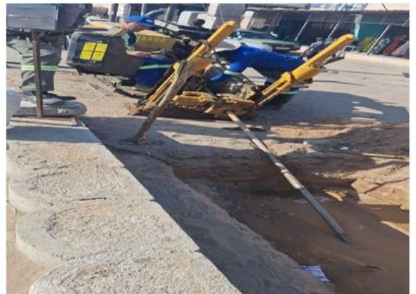
Pipe Installation of HDD
