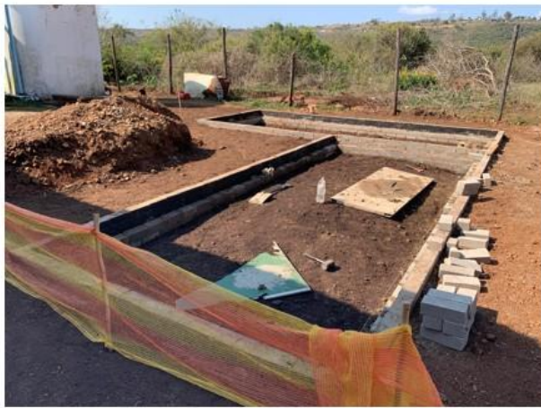
Preparation for concrete Slab -Staff Compound
