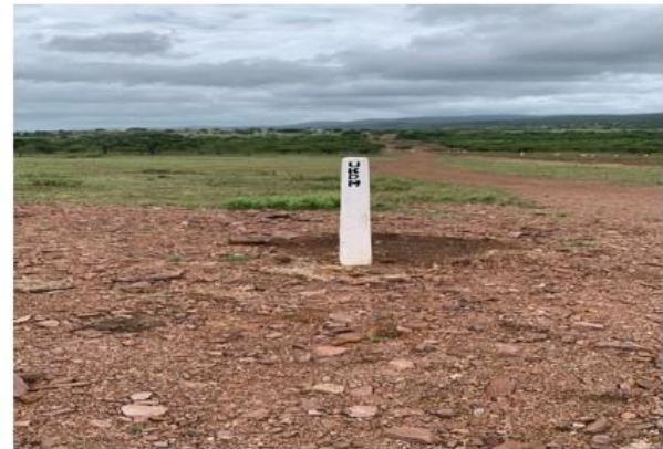
Pipe Markers for completed pipeline
