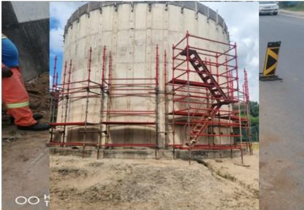
Scaffolding erection in progress
