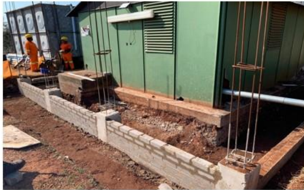
Pumphouse Foundation-In Progress
