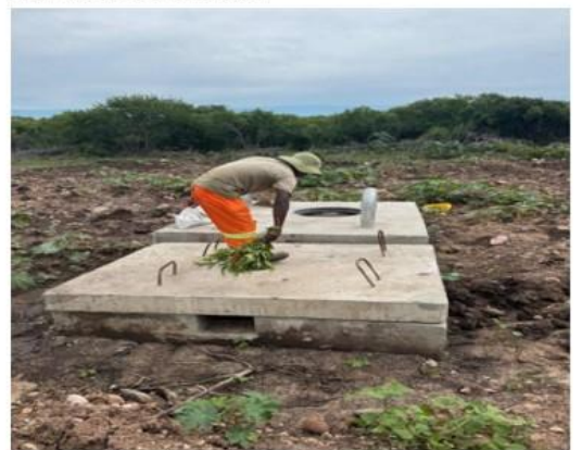
Air Valve chambers with complete Rehabilitation
