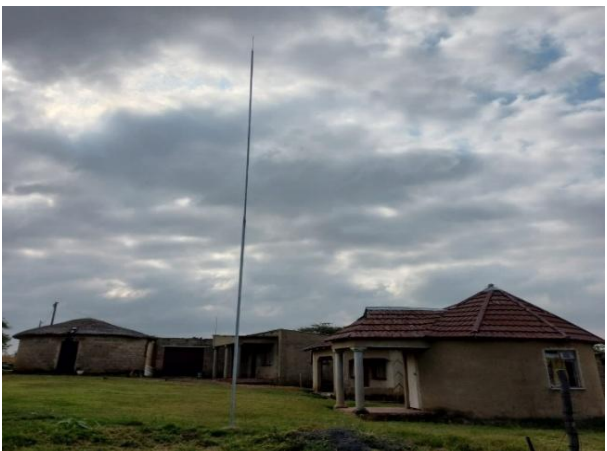
Lightning conductor installed at Wasbank in ward 1 at Endumeni
