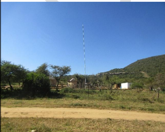
Lightning conductor installed at Muden in ward 11 at uMvoti
